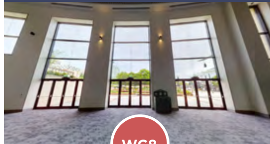
MLK Lobby North above doors
